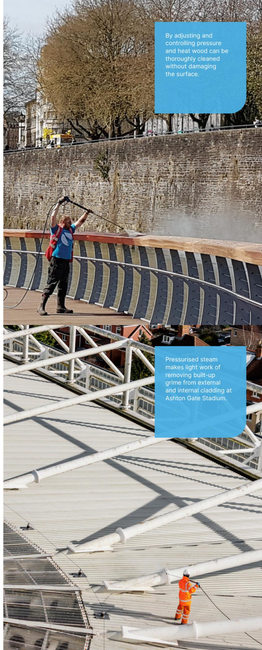
By adjusting and controlling pressure and heat wood can be thoroughly cleaned without damaging the surface.
